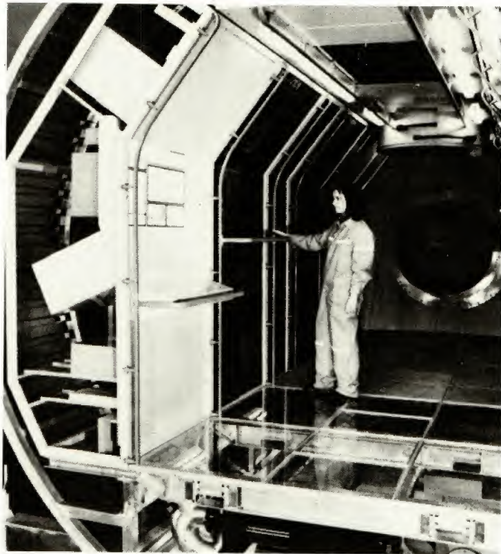
LAB Module during construction.
